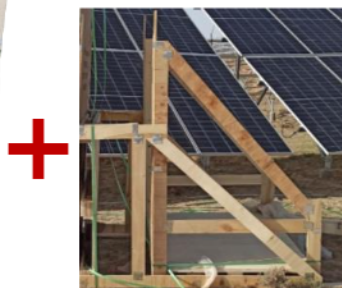
Support with wooden bracket
