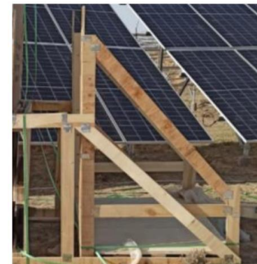
Simple anti-tipping bracket
